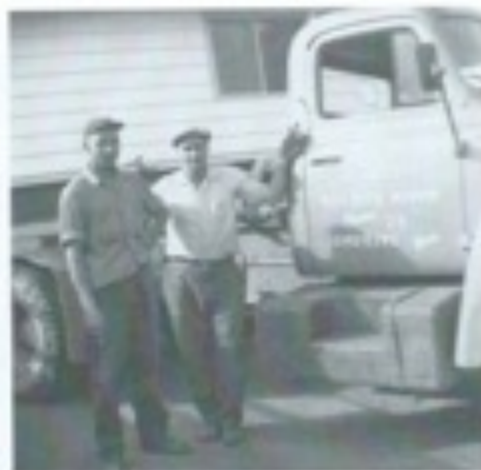
July 1963 Marcol Perini building moved from Somerset MS.
